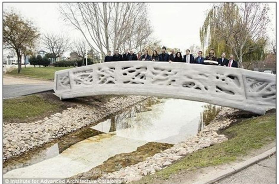
The Institute for Advanced Architecture of Catalonia has designed the first 3D printed bridge in the world
